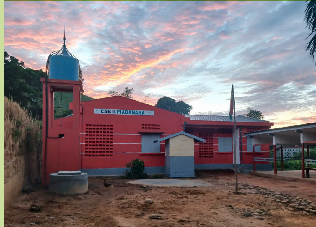
The Fiadanana Health Center, newly renovated in partnership with Fondation AXIAN.
